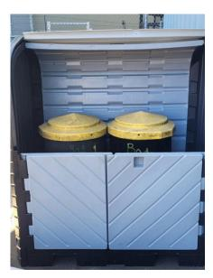
Pictured above are, left to right, the company's outdoor used oil storage area before and after installation of a covered shed which contains an internal spill pallet. The unique design of the shed ensures the areas rain water runoff is not contaminated by the residue oil from the drums and the floors "drip pan" design easily contains any unexpected spillage which may happen while transferring oil into the drums.
