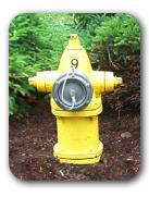
Fire Hydrants are a critical part of fighting fires in our communities. Fire hydrants are connected to our water distribution systems, a network of underground pipes. Therefore, the water that comes out of a fire hydrant is the same drinking water used in our homes, businesses, and schools. Fire hydrants in colder climates, such as our area, use "dry barrel hydrants" which
