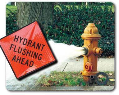
valves, one section of main at a time, to force the water through the pipes at high velocity, removing accumulated mineral sediment until the water is clear.
