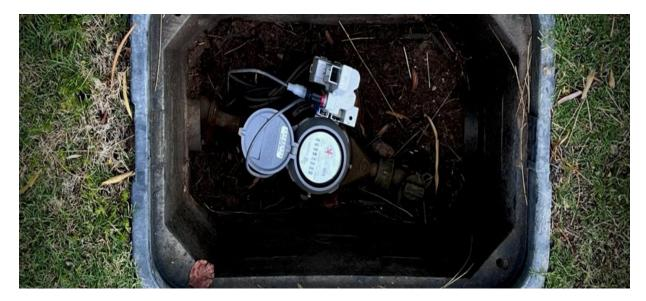
**Note:** Your meter reads in cubic feet. One cubic foot equals 0.748 gallons. If you determined that 100 cubic feet were used during a meter test, then 74.8 gallons were used. All you must do is multiply the cubic feet by 0.748.
