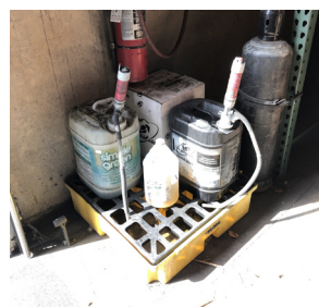
1. Spill containment pallets
