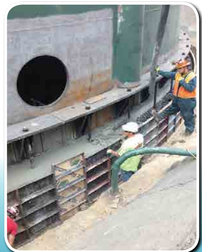
Pouring concrete in the support foundation at the View Acres water reservoirs seismic upgrade.
