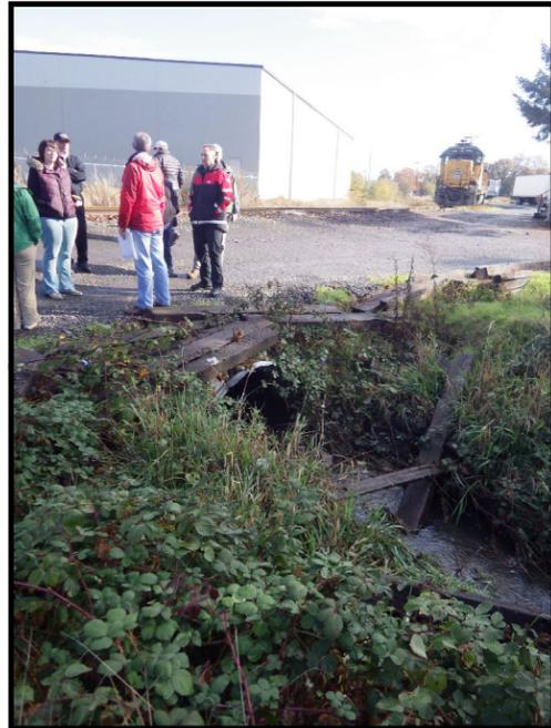
Photo B. Stormwater outfall to Cow Creek.
