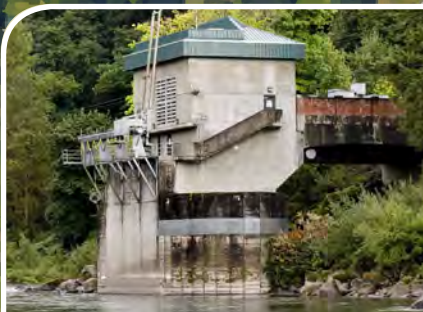
Drinking Water Intake Facility
